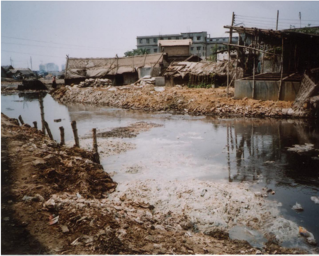
Photograph -12: Fleshings & other Solid Wastes reducing the carrying capacity of Hazaribagh_Canal near Kalunagar at Hazaribagh
