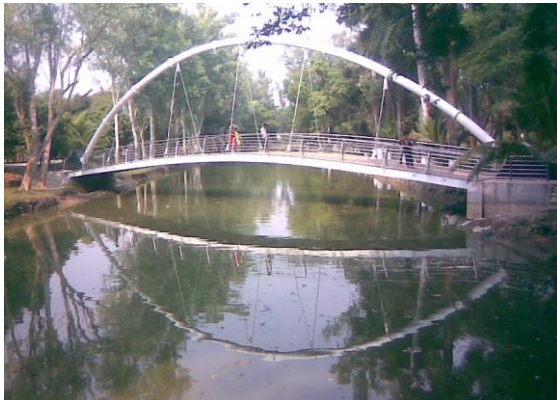
Foot over bridge on lake
