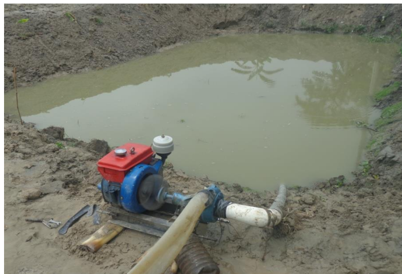
Plate 3.5: Pond excavation in the study area
