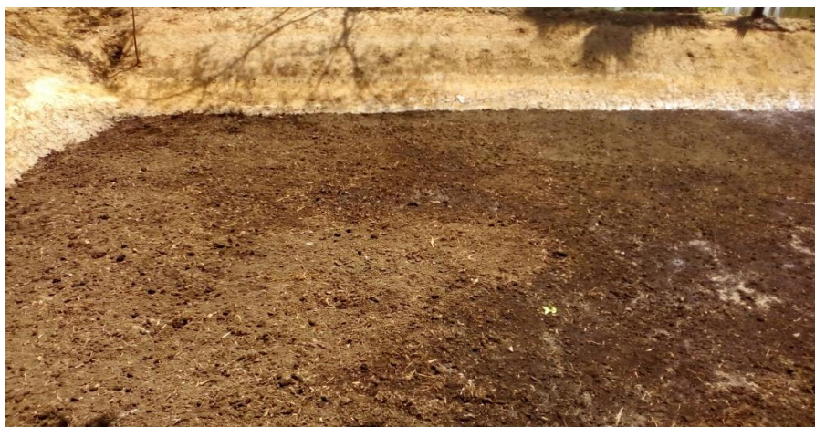
Plate 3.8: Pond excavation in the study area
