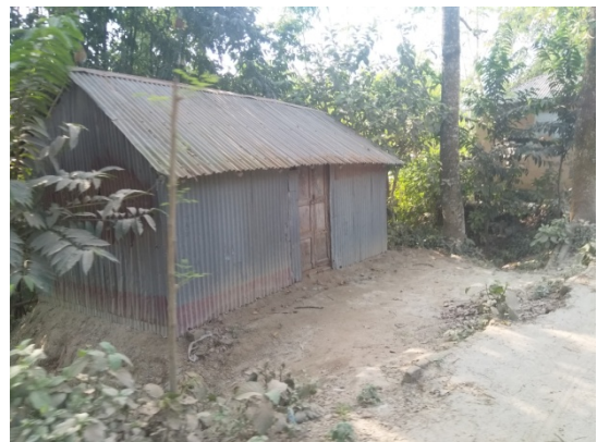
Embankment side settlement
